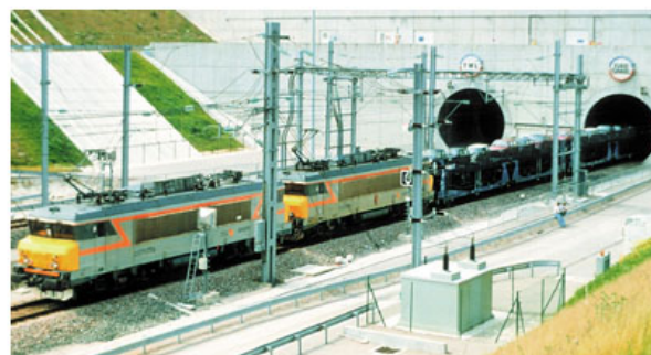
In operation: high speed railway tunnel Eurotunnel France – Great Britain
