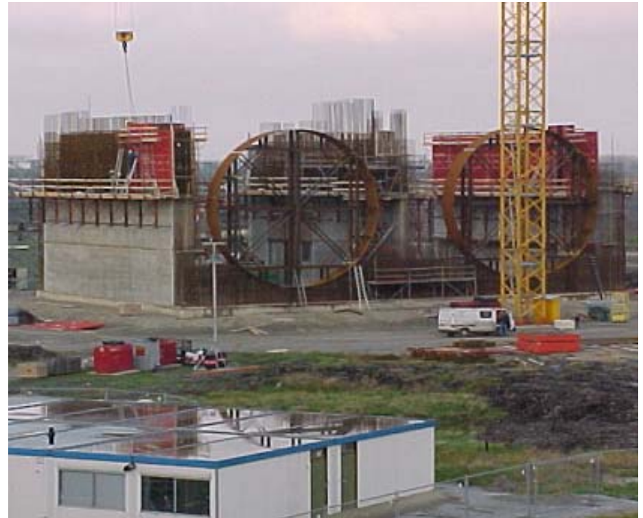
Target construction before lowering in position
