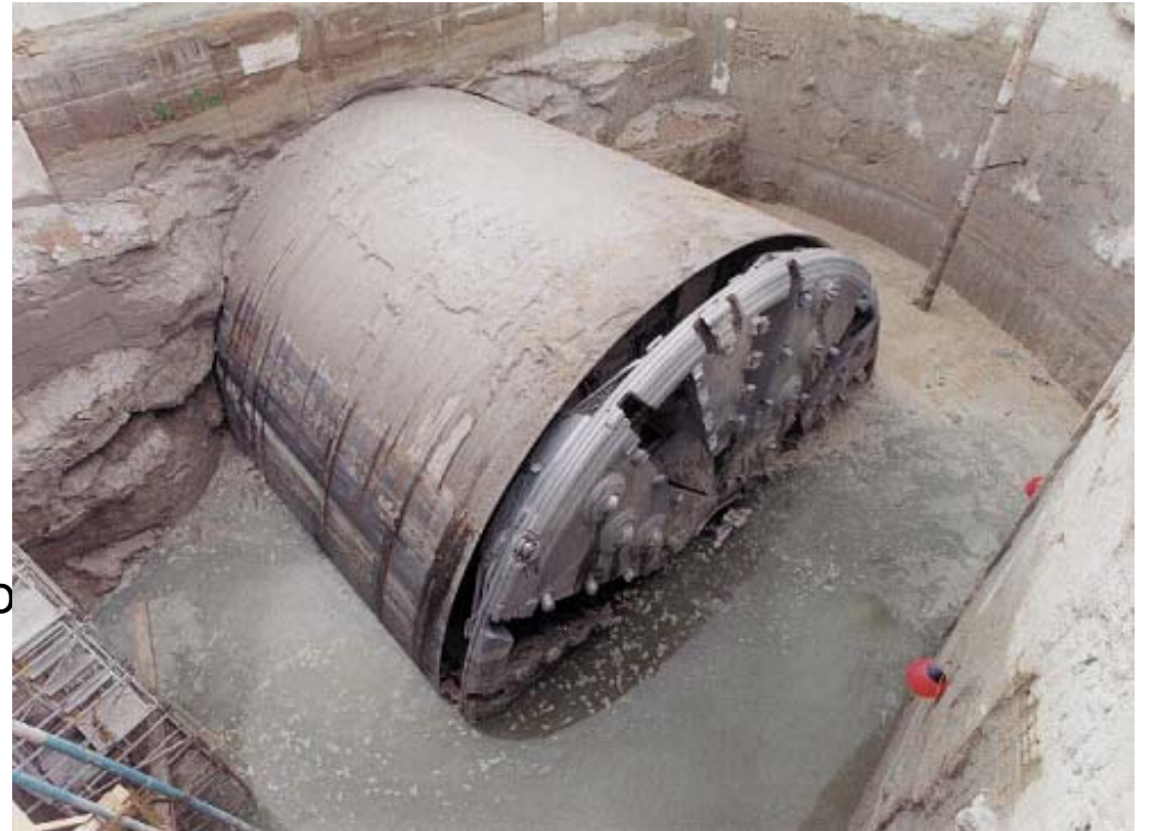
Seal against groundwater at Elbe Tunnel, Hamburg
