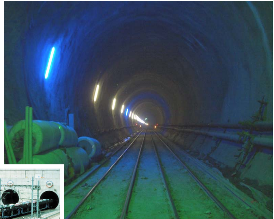
Under construction: high speed railway tunnel Alptransit Gotthard Base Tunnel (Switzerland)
